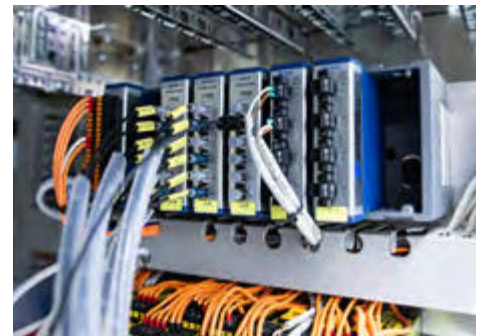
Figure 6: Time-precise control via fiber optic cables and analog measurement
